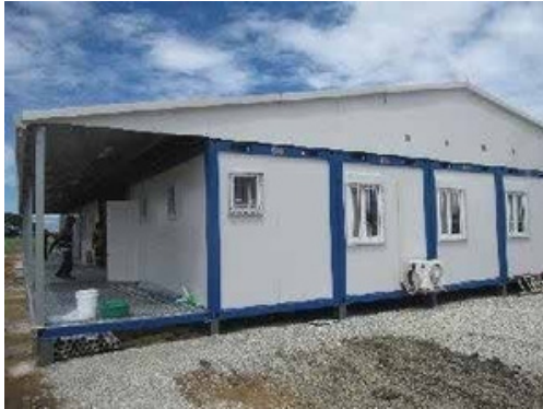
Construction Site Office
